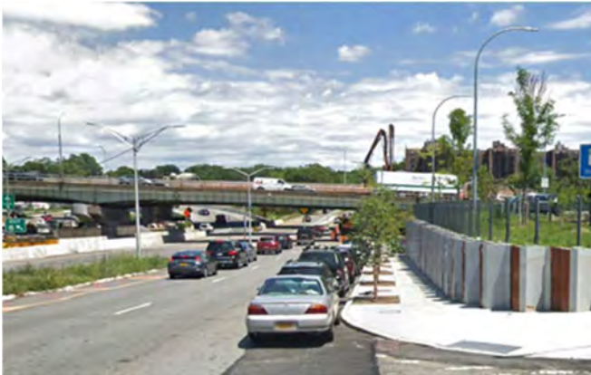
Figure 10. View north from Union Turnpike at 126th St.
