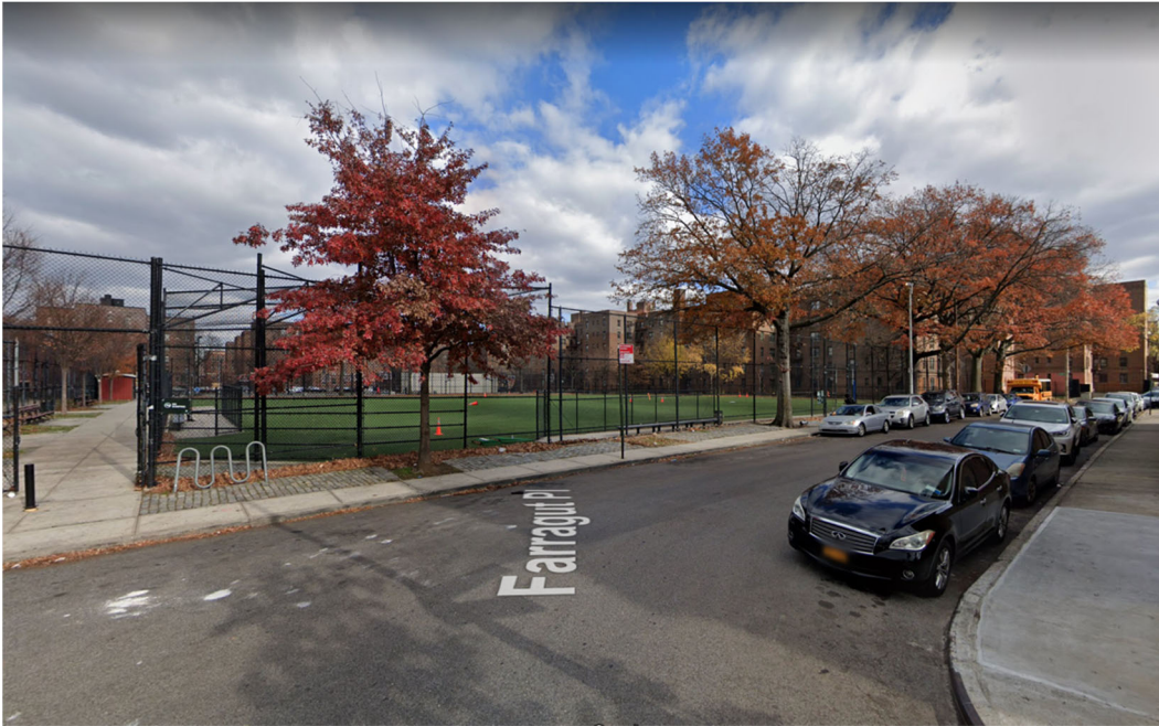
View of project site along Farragut Street, facing northwest
