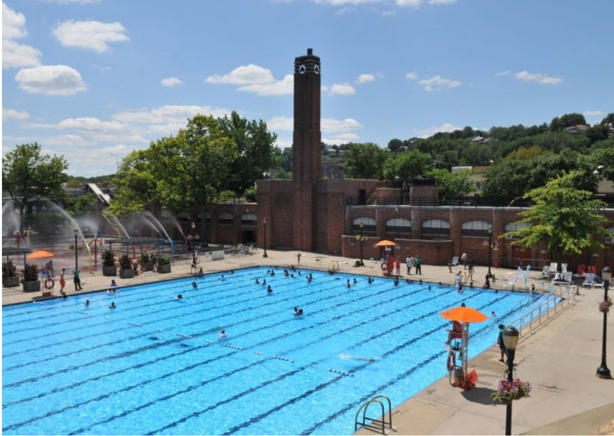
Lyons Bathhouse Facility, facing Southwest
