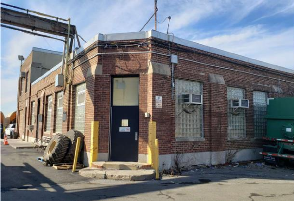
View of South East Corner of the Administration Building
