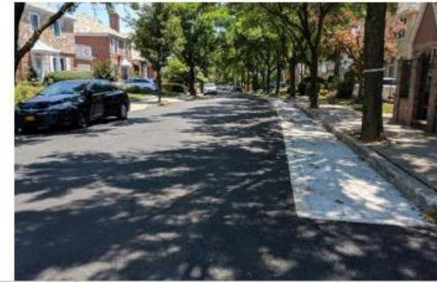
A FINISHED POROUS PAVEMENT INSTALLATION IN QUEENS.
