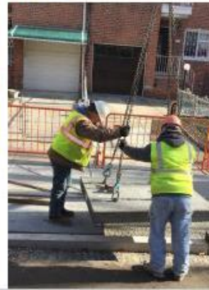
CONTRACTORS INSTALL POROUS PAVEMENT IN THE ROADWAY
