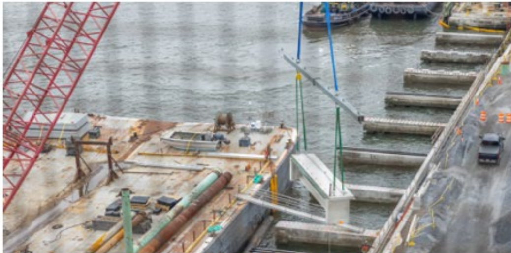
Prefabricated esplanade support beams being place, January 2024
